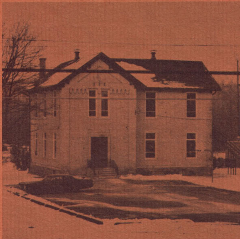
EBERSOLE COMMUNITY CENTER (formerly California Grade School — Erected 1870)
